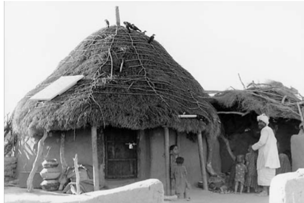
Figure 12. Typical solar home system (Rajasthan, India).
